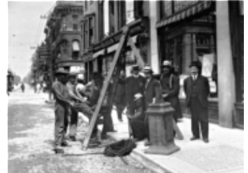
AFC 341-S4-SS1-I12 Electrification - crew working next to E.V. Buchanan. -- 1911. -- 4x5 copy negative. -- Box Number AFC 341-18
