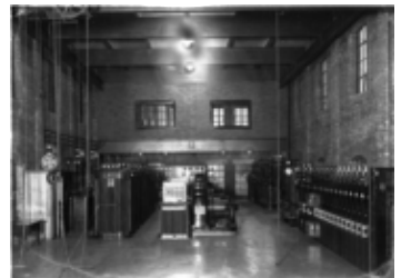
AFC 341-S4-SS1-I16 Horton Street Station - DC converters for streetcars. -- 1912. -- 6.5x8.5 glass plate negative. -- Box Number AFC 341-4 AFC 341-18
