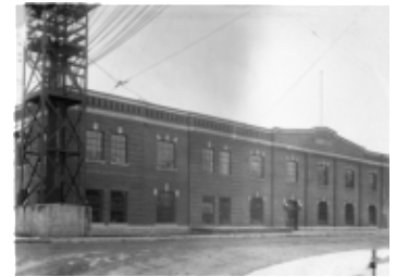
AFC 341-S4-SS1-I32 No. 5 Substation street railway and radials. -- 1910. -- 6.5x8.5 copy of glass plate negative. -- Box Number AFC 341-18
