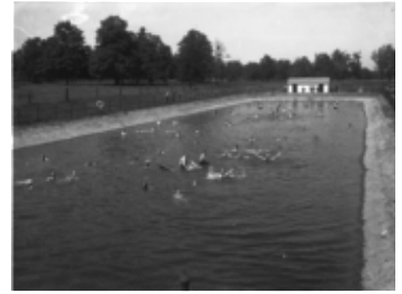
AFC 341-S4-SS2-I8 Outdoor swimming pool. -- [192-]. -- 6.5x8.5 copy of glass plate negative. -- Box Number AFC 341-18
