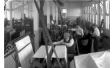
AFC 341-S8-I19 Luxite Textiles factory interior 2. -- 1920. -- 6.5x8.5 copy of glass plate negative. -- Box Number AFC 341-19
